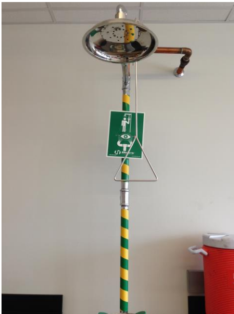
Figure 8: Shower & Eye Wash Station, Shower Instructions
